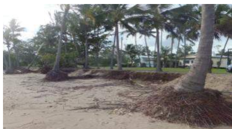
Before sand scraping
